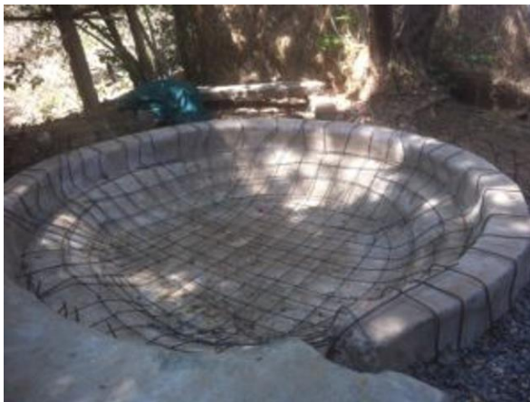
Figure 5 & 6: Building mesh structure
